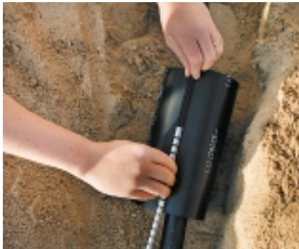
2 Sleeve is positioned over splice or damaged area and closed with metal channel.
