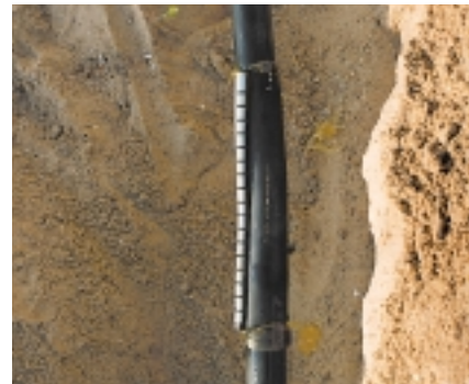
4 Finished sleeve is moisture resistant and durable.
